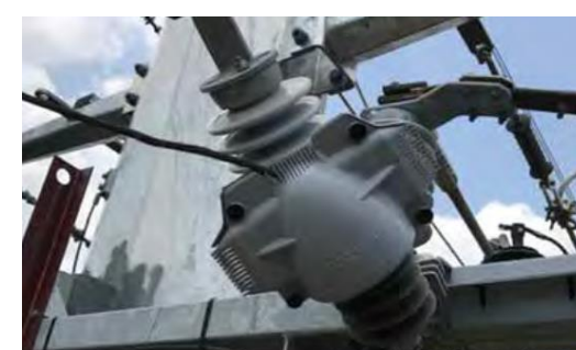
LIGHTNING ARRESTER GUARDS
