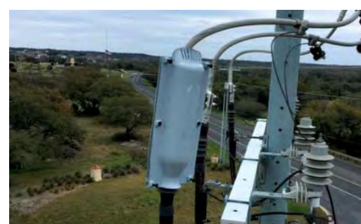
CABLE TERMINATOR GUARDS
